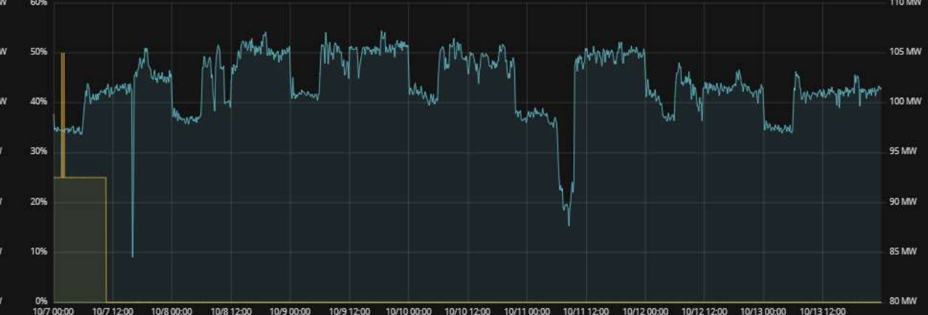
Chiller2 (Compresores/Free Cooling)
